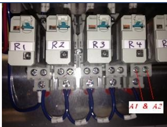
Detail 2 – Monitor relays, terminals A1 & A2
